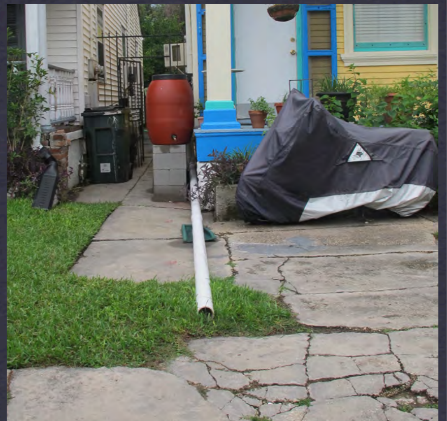
DUBLIN STREET :: FLOOD UNDER HOUSE NO MORE :: NOLA BAMBOO TWO 55-GALLON BARRELS WITH DIVERTER, CATCH BASIN AND EXTENDED DOWNSPOUT
