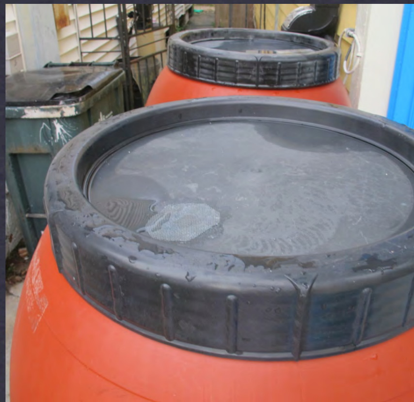
DUBLIN STREET :: FLOOD UNDER HOUSE NO MORE :: NOLA BAMBOO TWO 55-GALLON BARRELS WITH DIVERTER, CATCH BASIN AND EXTENDED DOWNSPOUT
